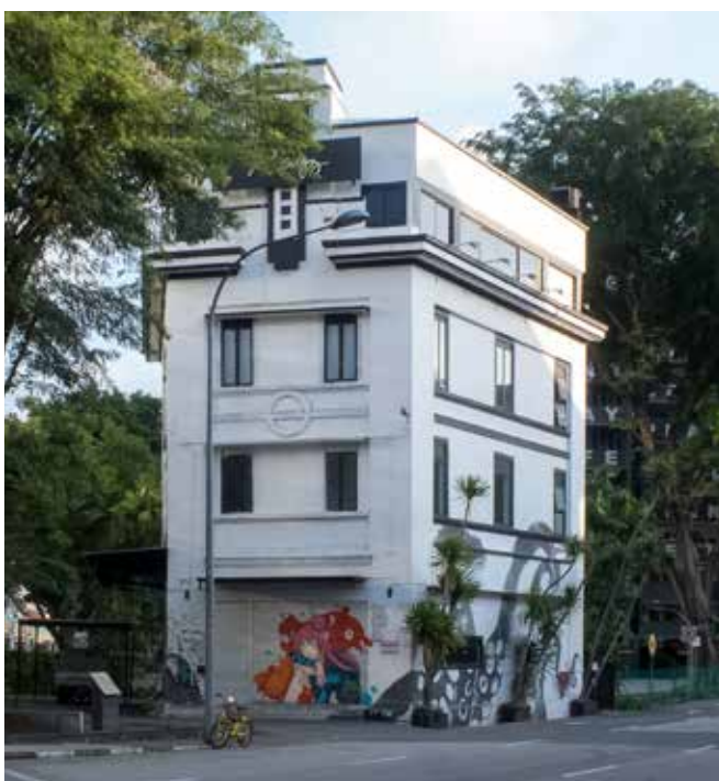
The building just before its demolition
